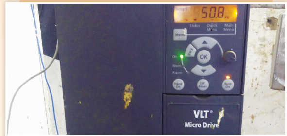
VFD installation at refrigeration compressor motor
